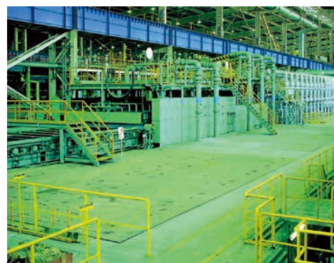
Heat treatment system
